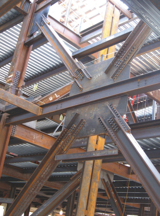
The hospital uses 13,000 tons of structural steel, including a 150-ft-long, three-story truss. Photos: Midwest Steel
