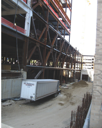
The hospital uses 13,000 tons of structural steel, including a 150-ft-long, three-story truss. Photos: Midwest Steel
