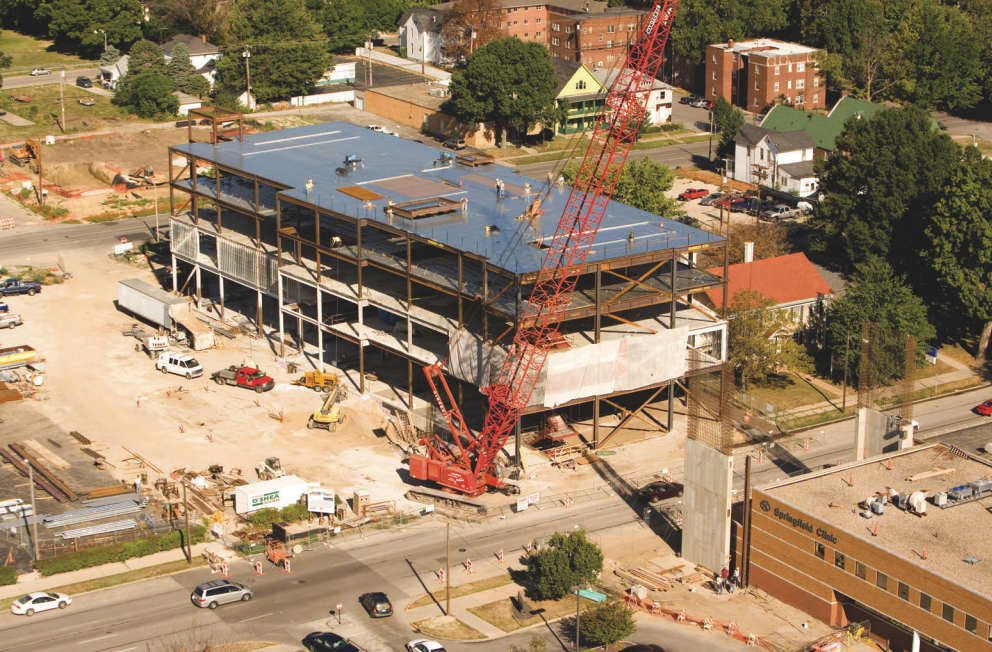
Hanging the curtain wall from the roof structure minimized the vertical movement under applied live loading and eliminated the need for expansion joints between levels.
